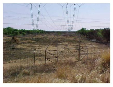
Figure 4 A game fence as used on the Matimba-Spitskop 1&2 lines. Note that the top section has been omitted as per the latest 5m game gate design.
